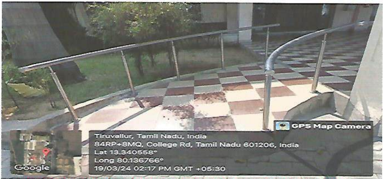
RAMP WITH RAILS FOR DIVYANGJAN IN ANNEXURE BLOCK
