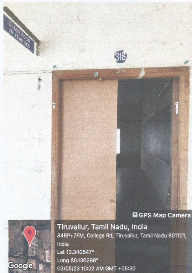
Room No. 318 - Front View
