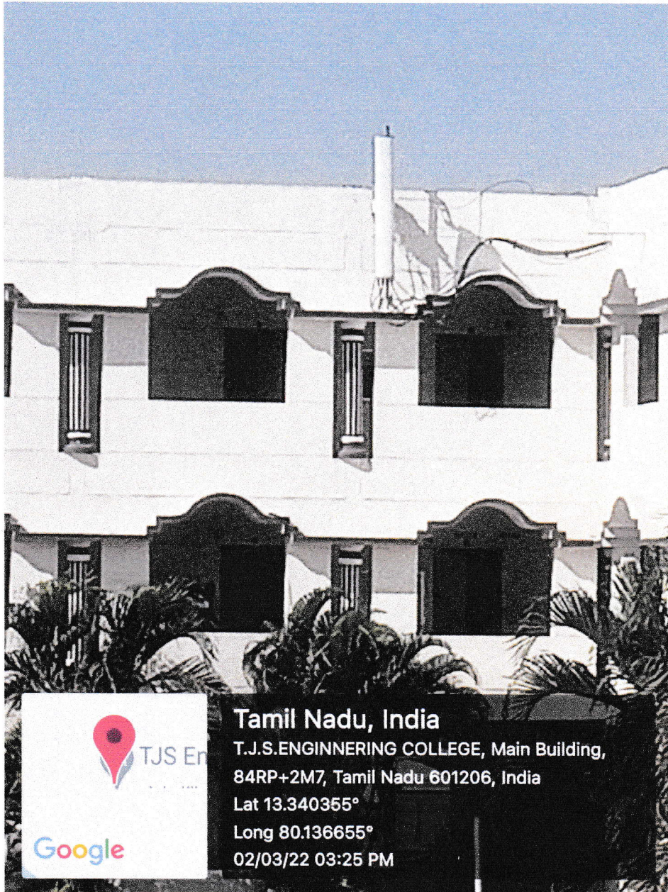
Bandwidth line placed inside the college campus.
